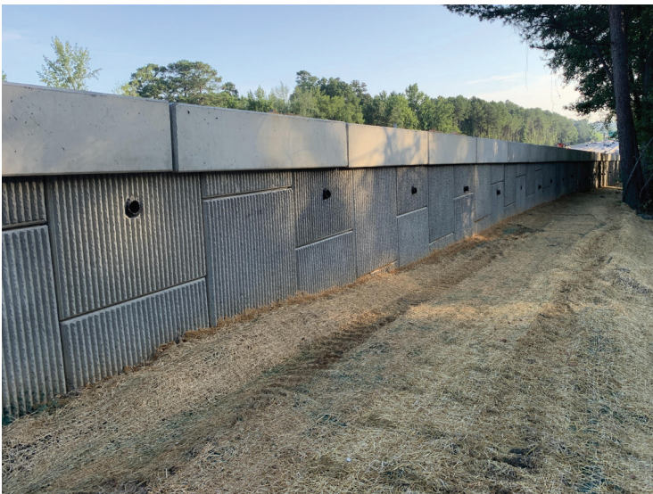
First completed MSE wall between I-26 westbound and McSwain Drive
