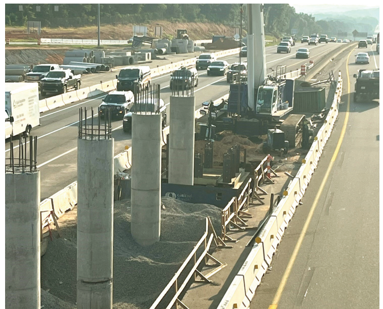
Bridge foundations being prepared for concrete to be poured
