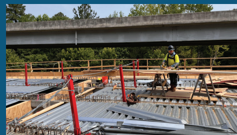
Carpenter building a frame during bridge construction
