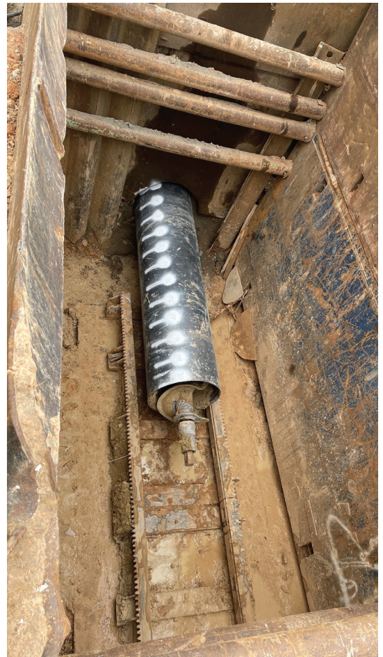
Jack and bore used in utility relocation
