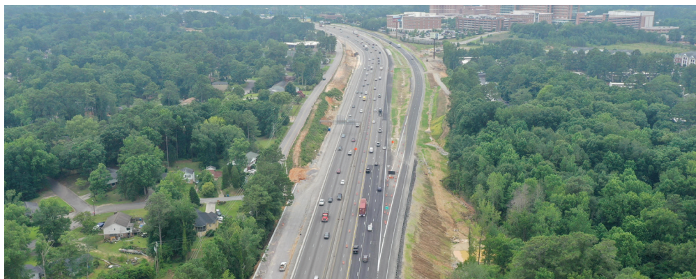
New exit ramp from I-26 eastbound to US 378, exit 110
