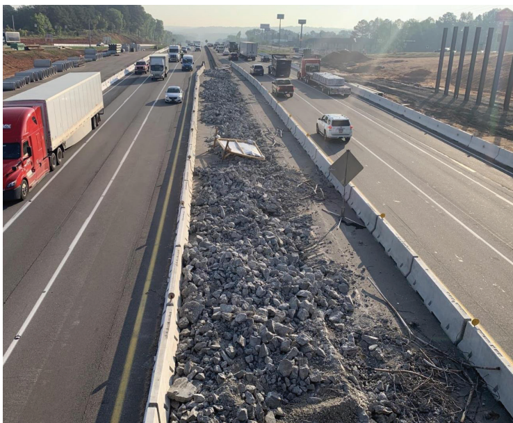
Demolition of median wall for the excavation of bridge foundations
