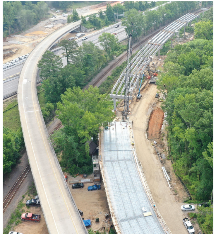
New bridge under construction near I-26 westbound to I-126
