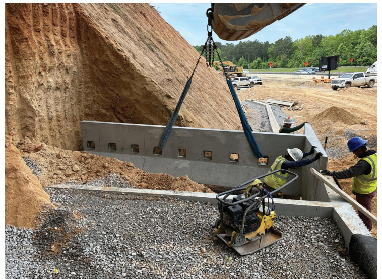
Crews installing Gravis retaining wall along I-26 westbound
